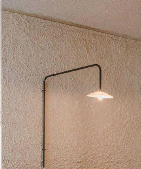
Stucco / textured finish then painted
